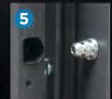
Anti-liftout frame pins
